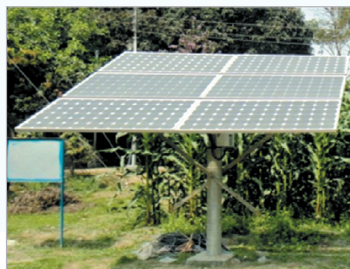
Fig. 3.12: Solar panel installed with fixed strong structure
